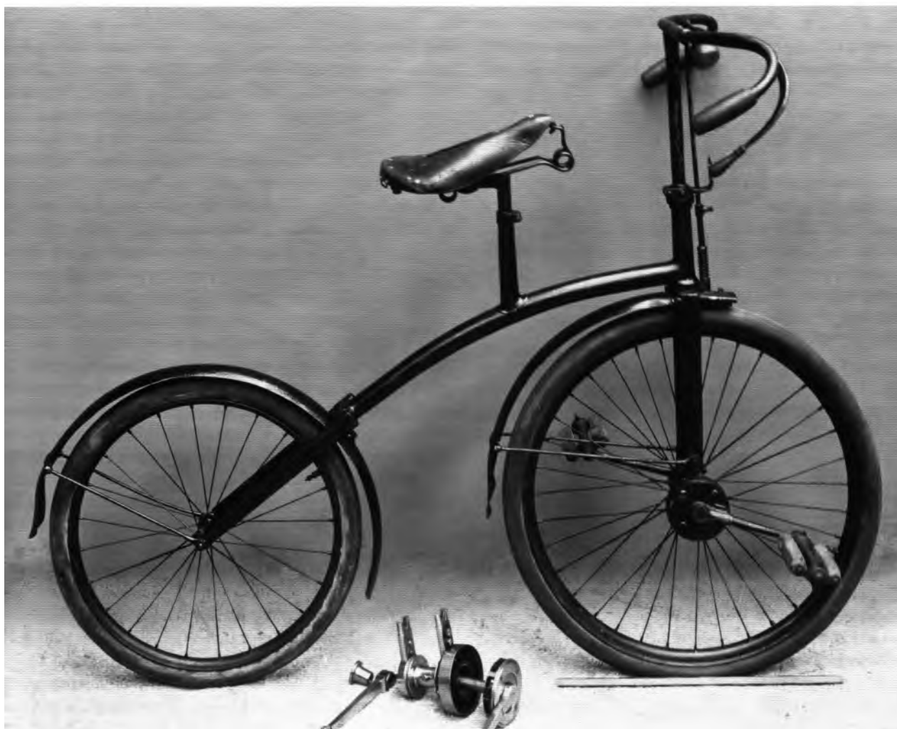
The 1893 Crypton featured a two-speed gear mechanism (front) and weighed about 13 kilograms (28 pounds). Today's road bikes can weigh as little as half that.
